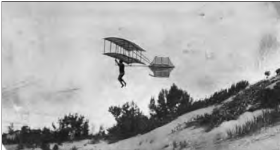
Octave Chanute understood the importance of wing shape for flight. In 1893 he wrote that “it seems very desirable that further scientific experiments be made on concavo-convex surfaces of varying shapes, for it is not impossible that the difference between success and failure of a proposed flying machine will depend upon the sustaining effect between a plane surface and one properly curved to get a maximum of ‘lift’.” National Air and Space Museum, Smithsonian Institution (SI 84-10696)
