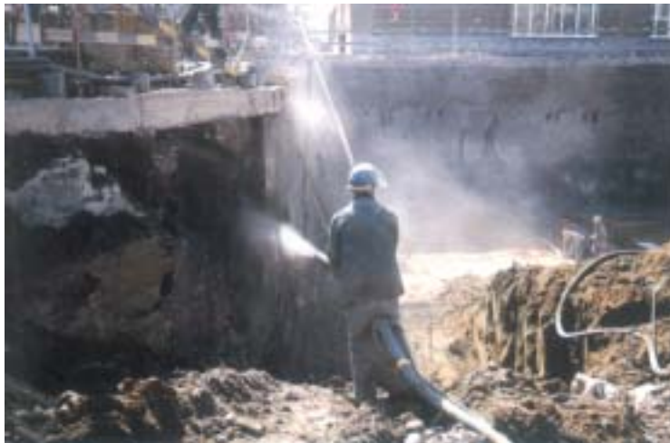
Steel wire fibre reinforced shotcrete
