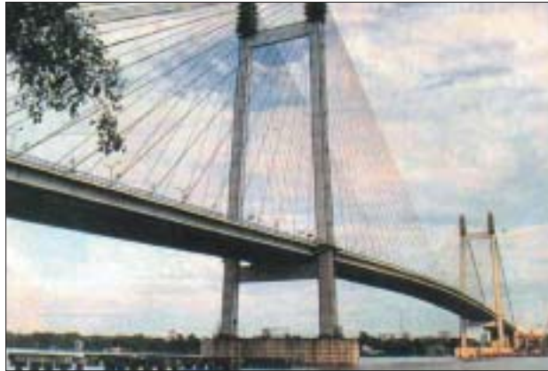
Vidya Sagar Setu at Kolkata where longest cable stayed bridge (in India) was built using high strength concrete.
