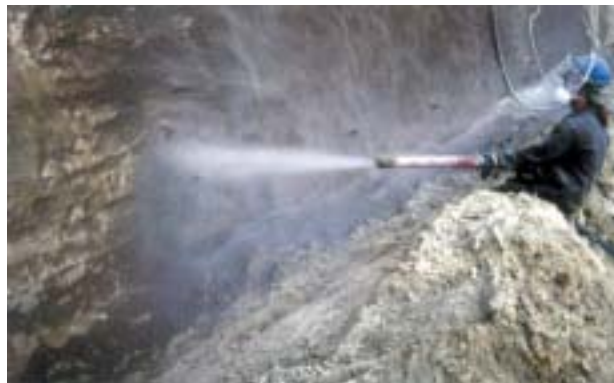
Shotcreting with steel reinforcement for slope protection.
