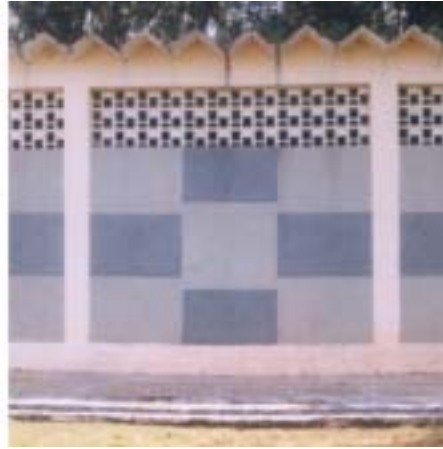
Ferrocement, "W" shaped folded plate roof for span 3.5 m. Thickness of plate is 20mm.
