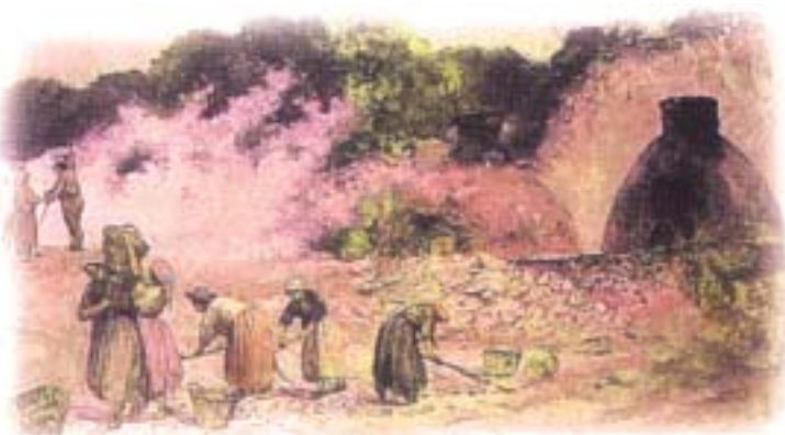
Joseph Aspdin's first cement works, around 1823, at Kirkgate in Wakefield, UK.
