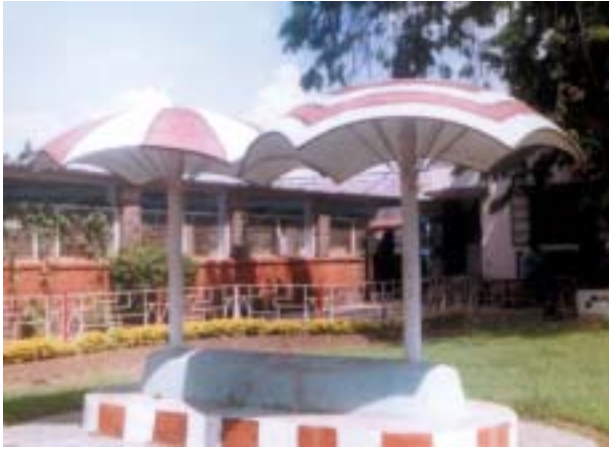
Ferrocement garden umbrella thickness 20 mm.
