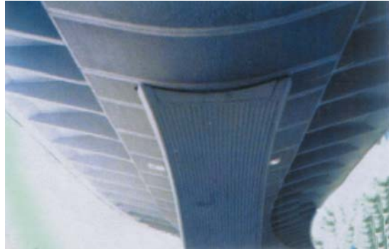
Acrylic based protective cum decorative coating is given to J.J Flyover at Bombay (shown above) and to many other bridges and flyovers in India, particularly in coastal regions.
