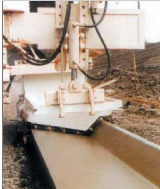
Mould with floating suspension for simultaneous casting of parapet wall.
