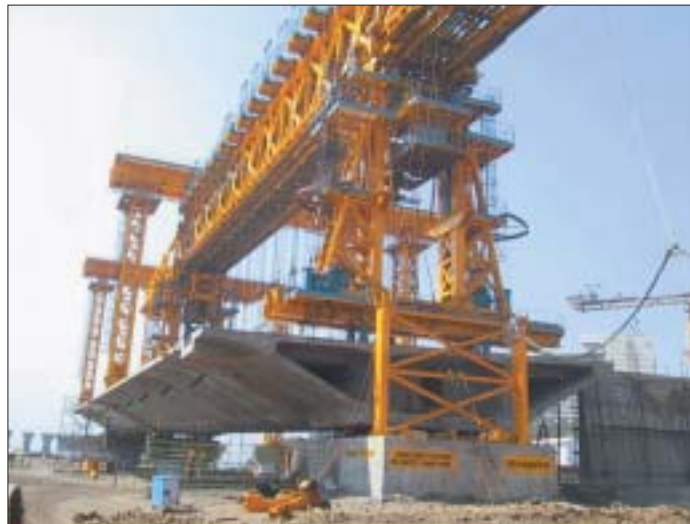
Bandra Worli Sea Link Project under construction with high performance concrete.
