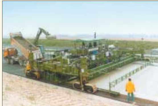
Fully automatic construction of concrete pavement.
