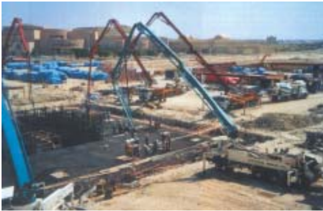
Concrete Pump and Placing Boom at Work in a Major Construction Site.
