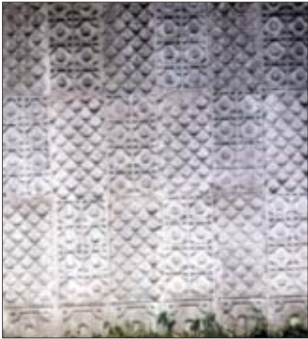
Applied finish work done at CME
