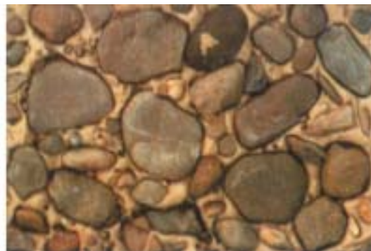
Badly pumpable concrete
