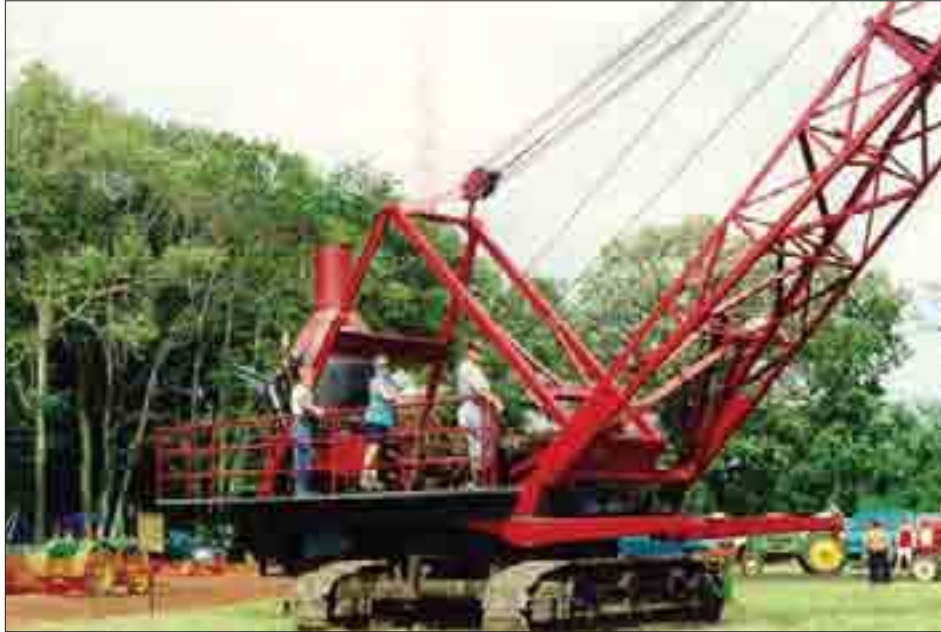
Ropes on a pile driver
