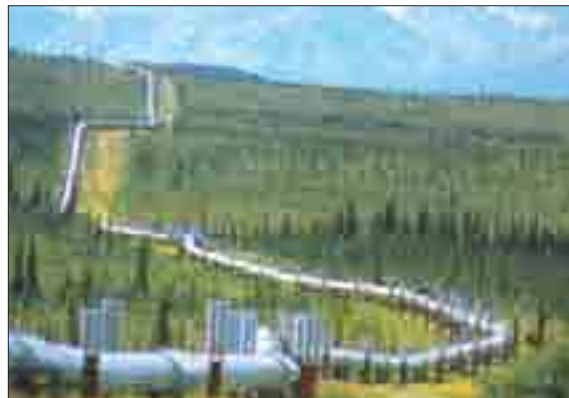
The Trans-Alaska Pipeline was built to carry oil across the frozen sub-Arctic landscape of North America.
