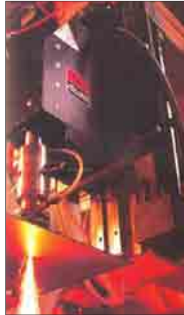
Lasers supported by computer controls can cut the metal very accurately
