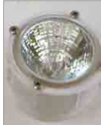
Retaining screws on a lamp.
