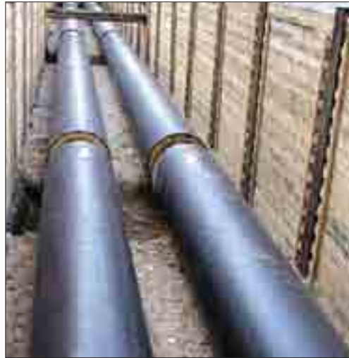
Cast iron pipes.
