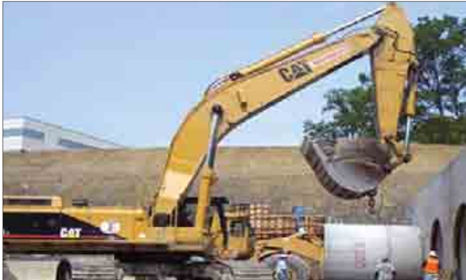
Excavator in action
