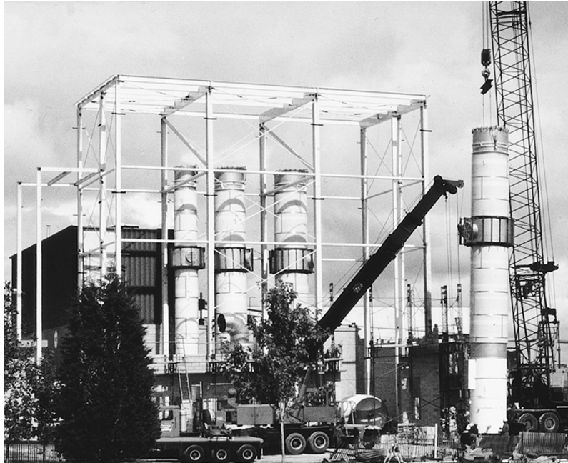
Fig. 12a. Multiple effect vertical tube evaporators (courtesy of APV Crepaco Inc.)
