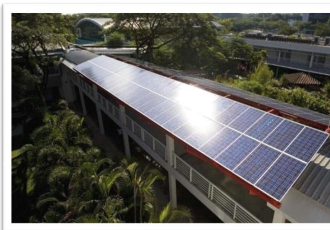
Fig-6 Solar pannels
