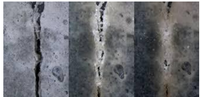
Figure-4: Before and after pictures of SHC's work
