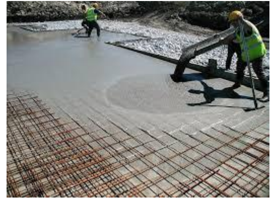
Figure-2: Pouring of SCC on slab
